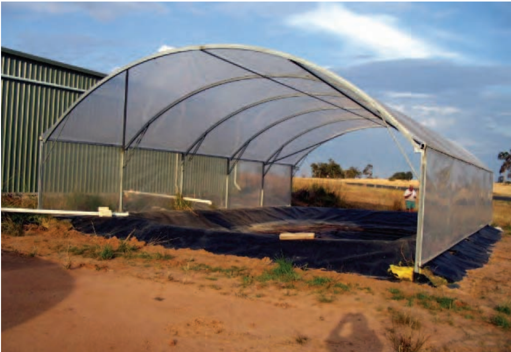
Plate 22. Evaporation pond with heavy plastic liner for the disposal of table olive wastewater. (Photo: Newton Ellaby and Merryl Ellaby, Australia.)
